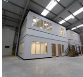
Warehouse Fit Out
